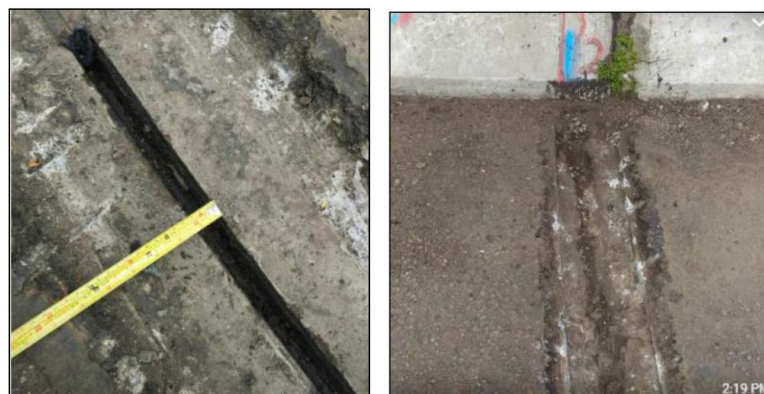
Gambar 4 Kondisi Expansion Joint P0 dan P1
