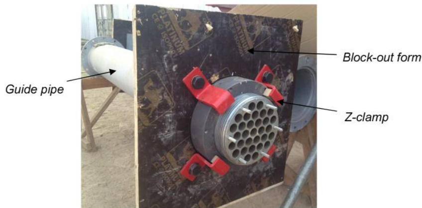
Gambar 12 Preassembly Angkur dan Recess Pipe
