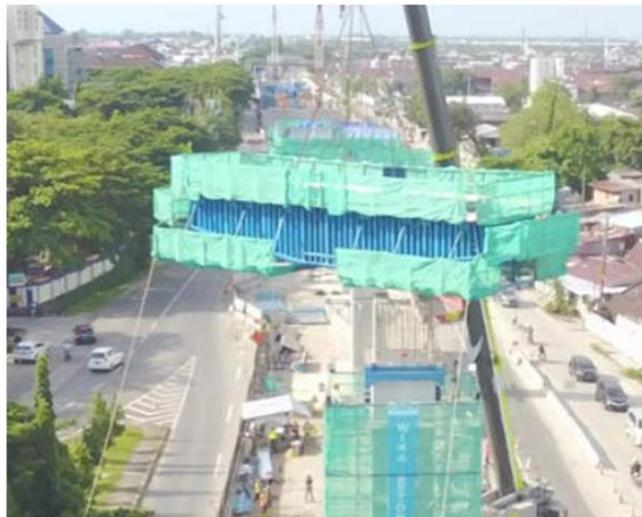
**Gambar 7** Metode Flying Pier Head Formwork System
