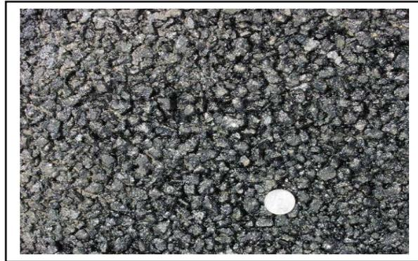
**Gambar 5** Perkerasan Beraspal Porus
