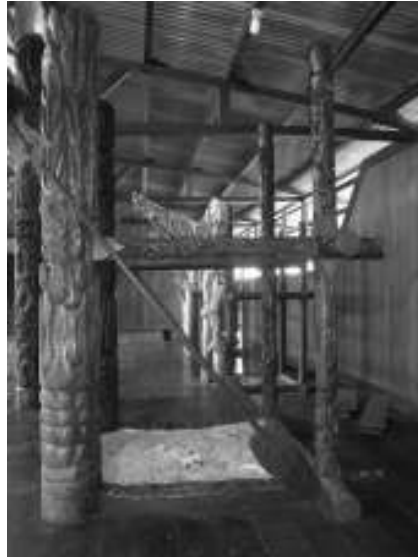
Plate 2. Fireplace and paddles in the Catholic Church of Sawa-Erma Parish, Asmat.
