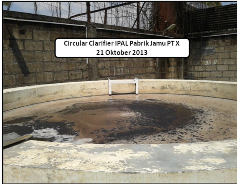
Gambar 5.1. Circular clarifier IPAL Pabrik Jamu PT X
