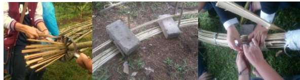
Gambar 0.3 Cold Bending Method: Bundling Technique
