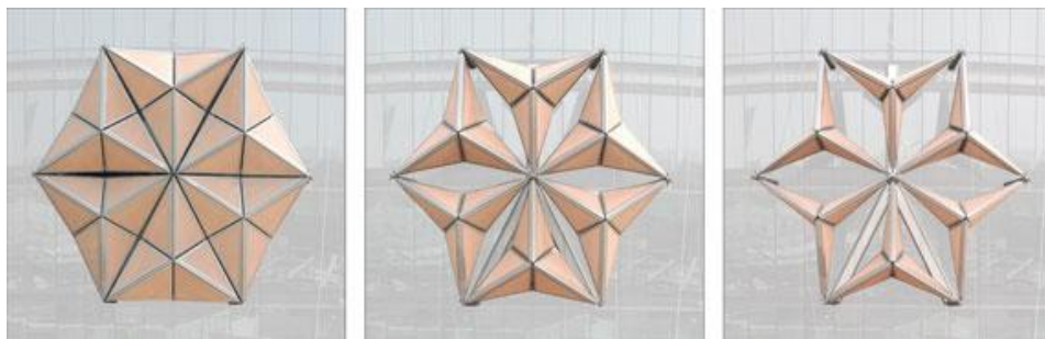
Gambar 4. Pergerakan Dynamic Facade Al Bahar, Abu Dhabi
