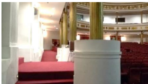
Figur 9. Pedestal kolom beton
