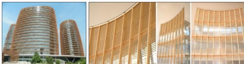
Gambar 1 Gedung Ruang kantor South Quarter dan Desain Fasad Louvre (Sumber: http://dienersyz.com/investments/ dan http://wkkarchitects.com/south-quarter-1/ )
