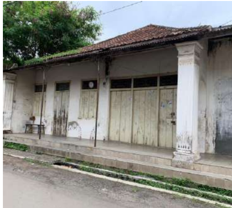
Figure 26 Front View of Building No.5 Residential Function
