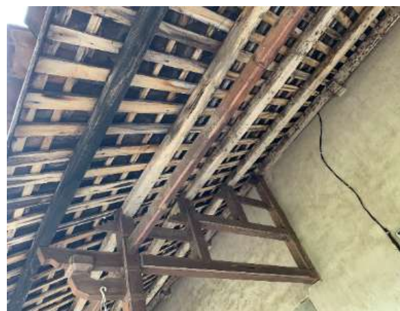
Figure 17 Dou Gong Shading Construction of Building No.2 Residential Function
