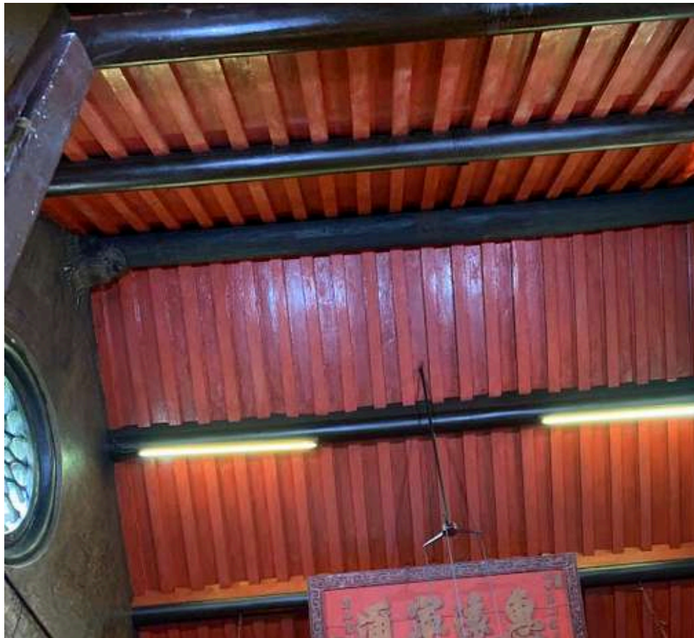
Figure 11 Teak Wood Wuwungan of Vihara Dharma Rakhita
