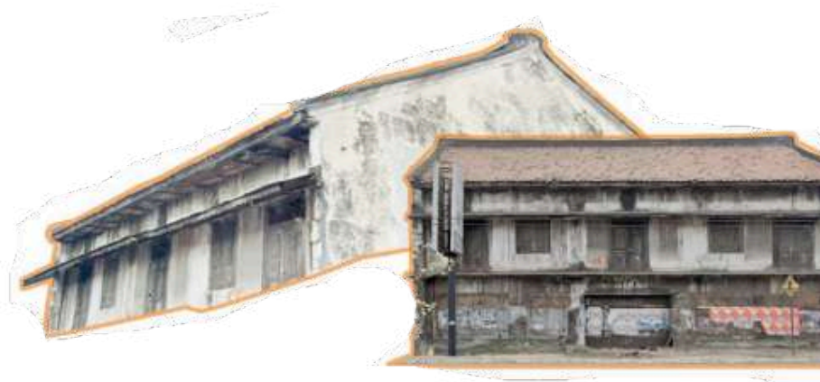
Figure 38 Front View of Building No.8 Residential Function Shophouse Type
